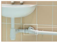
The non-return valve  $\emptyset$  50 in version A is fitted in the horizontal course of  $\emptyset$  50 sewage pipework attached to the wall by means of brackets.
