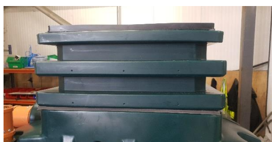
Figure 3: Single MDPE Riser fitted onto HC6 model
