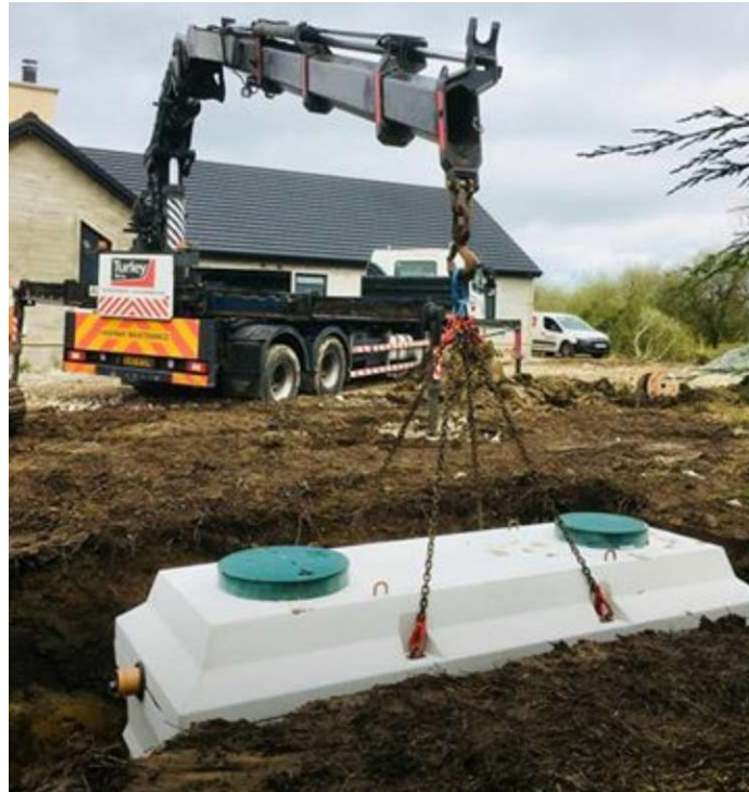
Position of lifting chains
